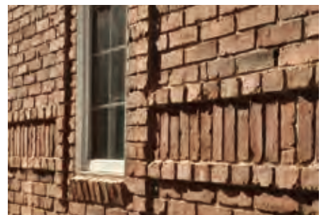
1-Half Brick Flat (半マス平) 3-Thick Half Brick Flat (半マス倍厚平) 7-Taper Half Brick Flat (クサビ型半マス平)
