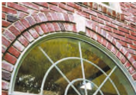
1-Half Brick Flat (半マス平) 3-Thick Half Brick Flat (半マス倍厚平)
