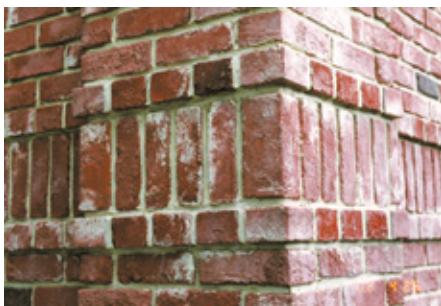
3-Thick Half Brick Flat (半マス倍厚平) 4-Thick Brick Corner (倍厚曲り)
