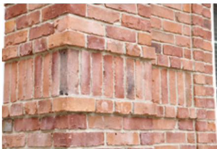
3-Thick Half Brick Flat (半マス倍厚平) 4-Thick Brick Corner (倍厚曲り)
